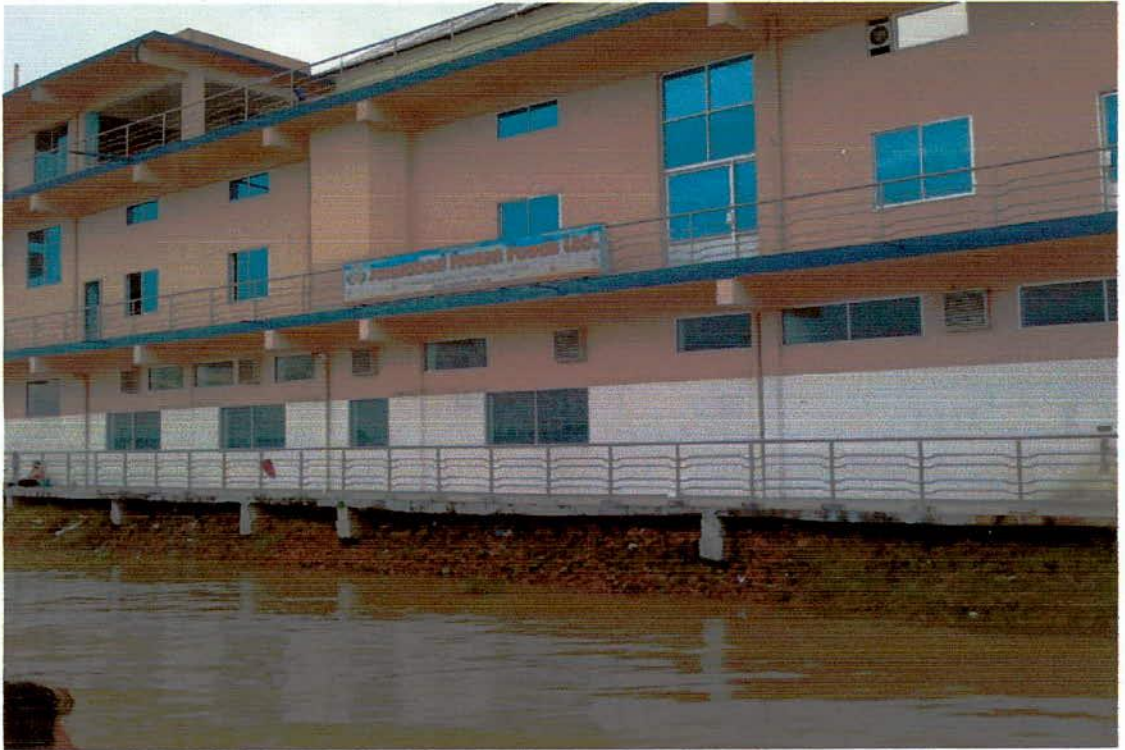
Fig 4.7: Sea food processing industry at Rupsha Bridge, Khulna
