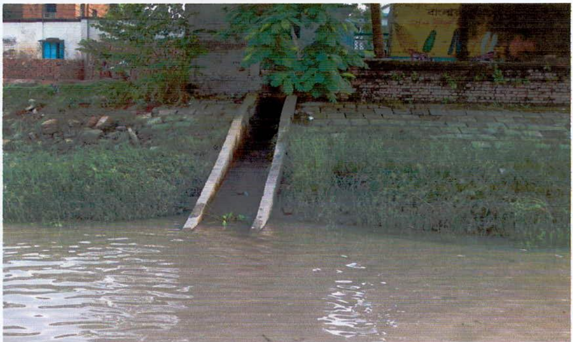
Fig 4.4: Municipal sewage at Kalibari Ghat, Khulna
