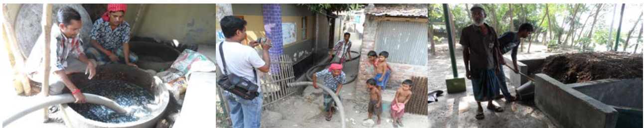
Figure 4.43: Emptying and processing without using any PPE
