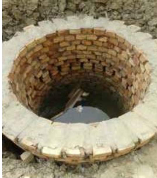
Figure 5.1: High level of underground water table
