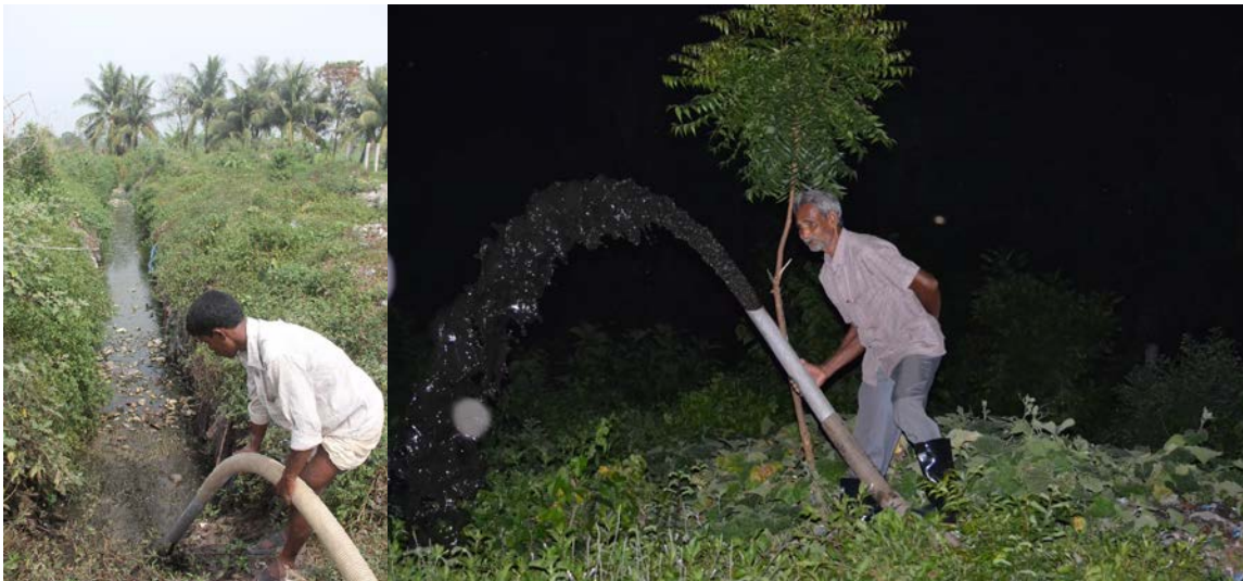
Figure 4.33: Trenching ground in Khulna City
