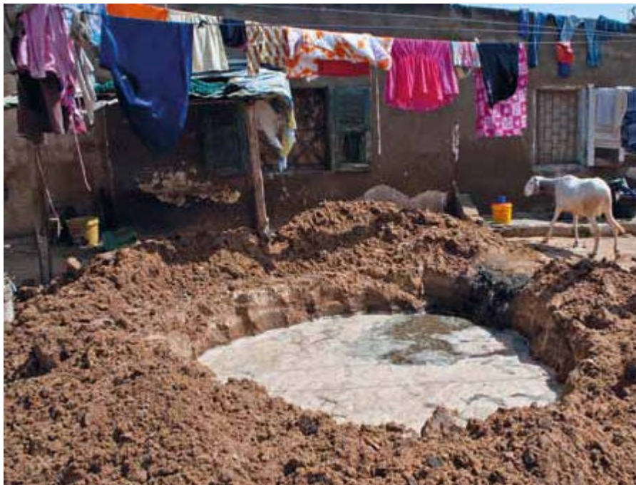
Figure 2.2: Faecal sludge from a septic tank next to the house in Dakar (photo: Linda Strande)
