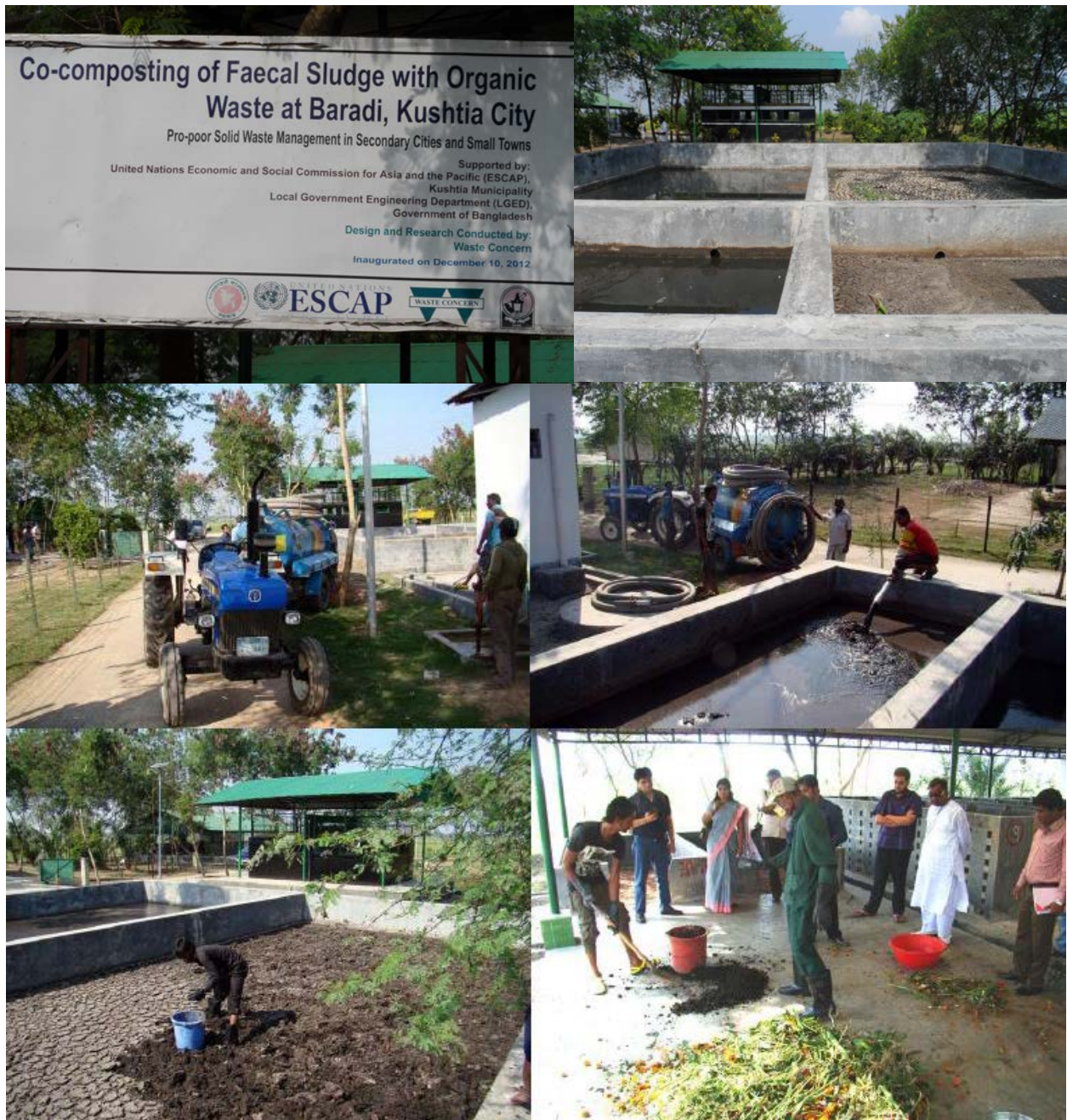
Figure 4.35: Drying Bed and Co-compost Plant of Kushtia Municipality
