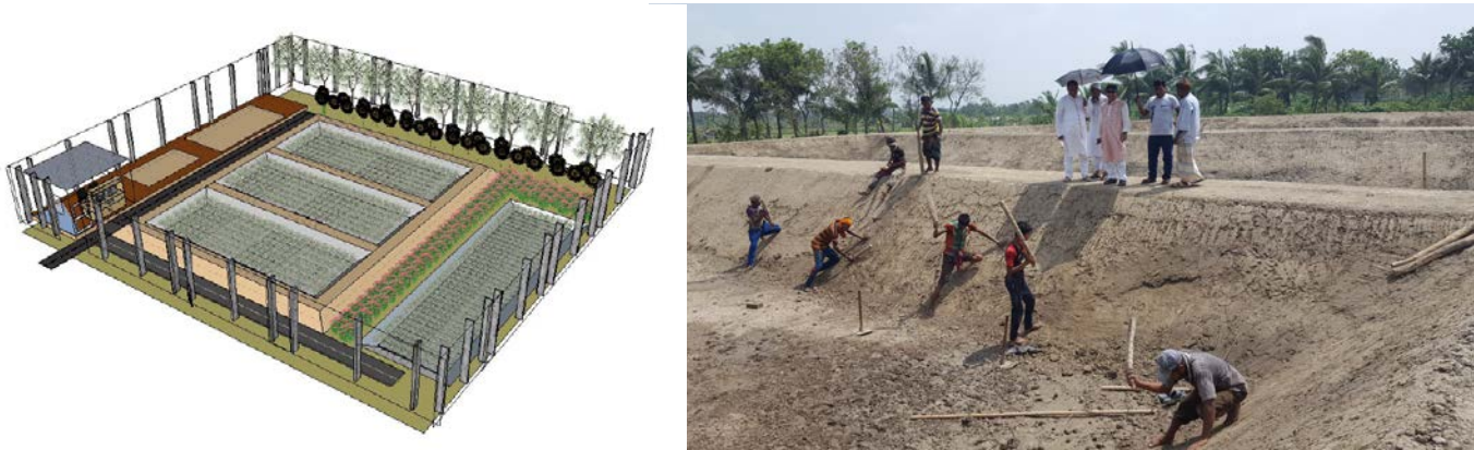
Figure 4.34: Construction of ongoing Constructed Wetland (CW) in Khulna
