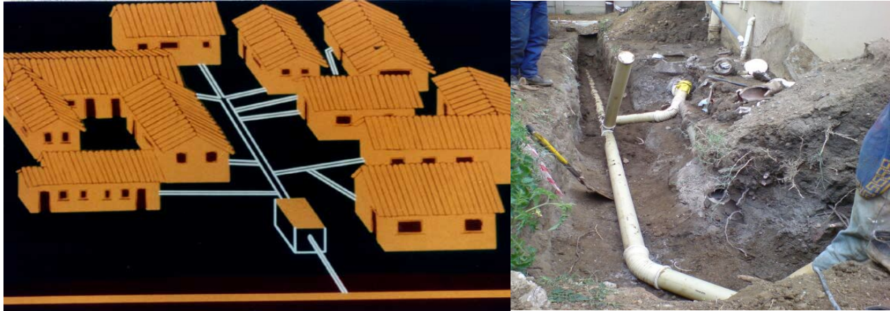
Figure 5.2: Small Bore Sewer (Source: https://www.google.com/small bore sewerage )
