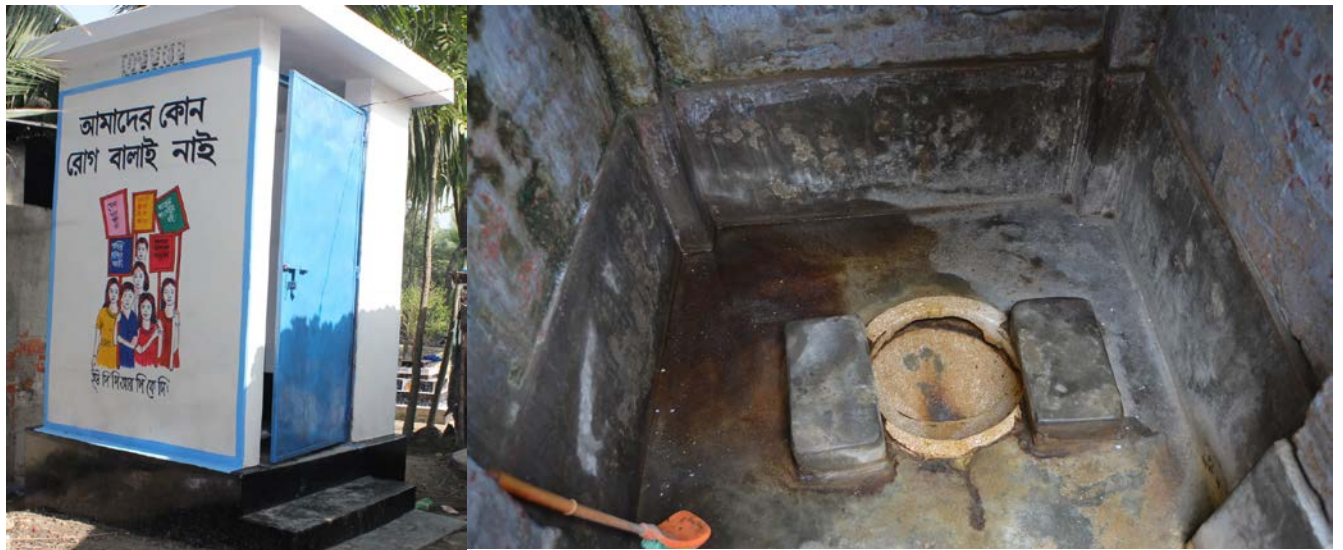
Figure 4.3: Pit toilet superstructure and inside condition in Kushtia
