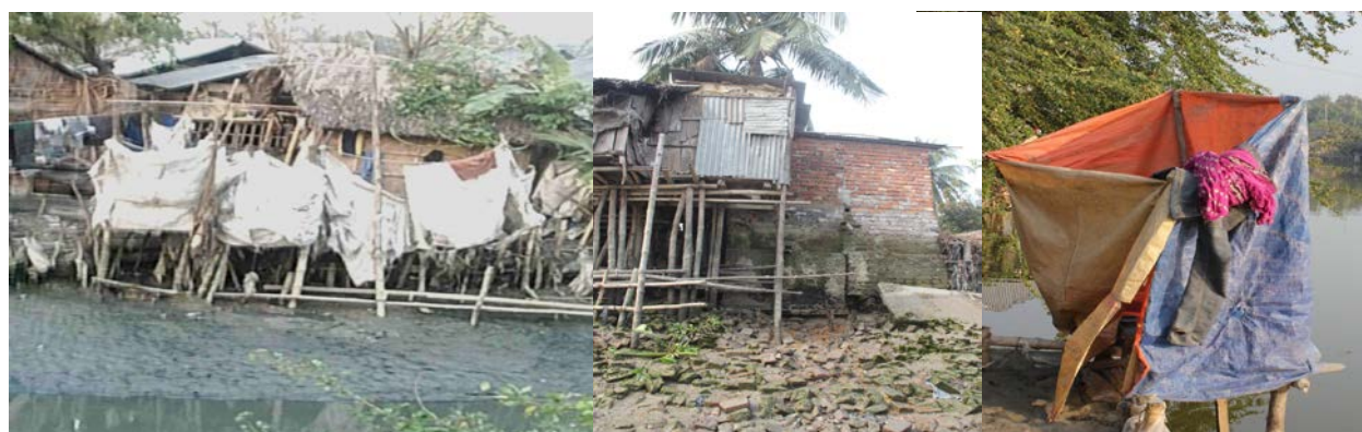
Figure 4.4: Hanging toilet in KCC
