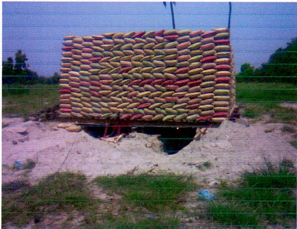
Fig-4.3 Static Pile Load Test
