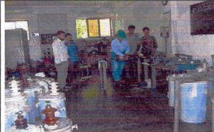
Picture-07: Technician are repairing distribution transformer
