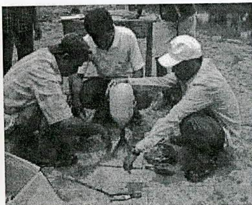
Figure 4.6 Field compaction test of the prepared CCL of the PSSL
