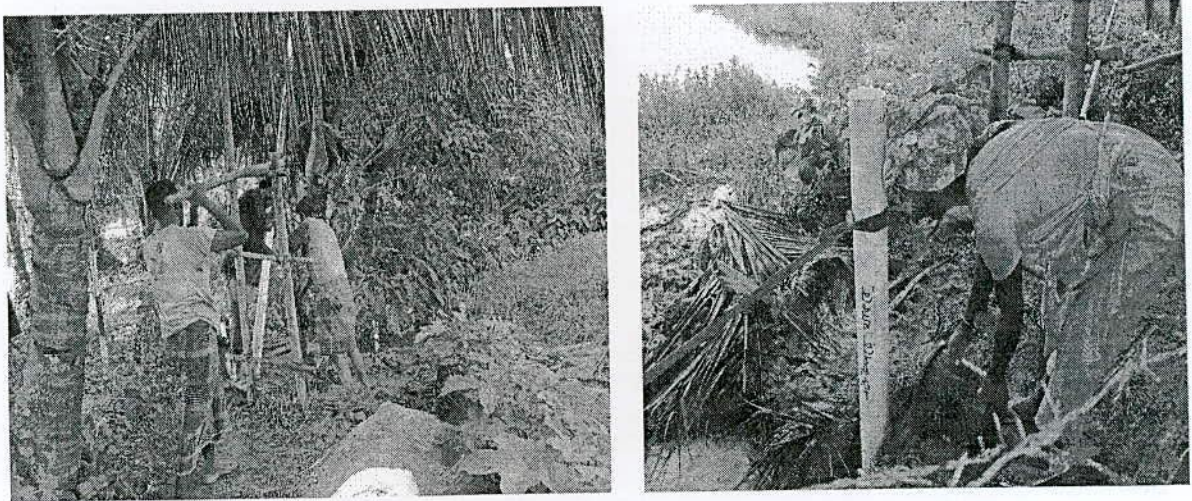
Figure 4.14 Construction of monitoring well in the pilot scale sanitary landfill
