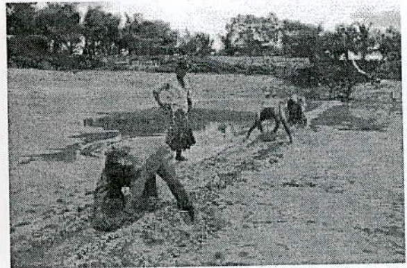
Figure 4.10 Preparation of bed to place leachate collection pipe
