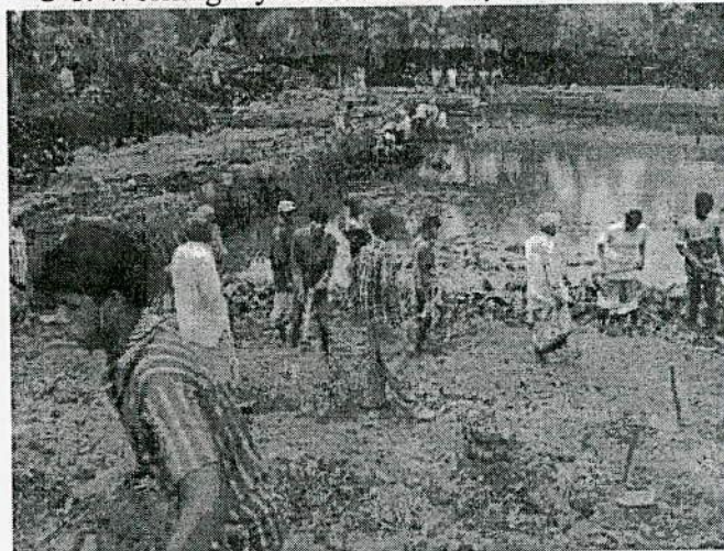
C-2. Earthwork in excavation of PSSL, dated 17.04.08
