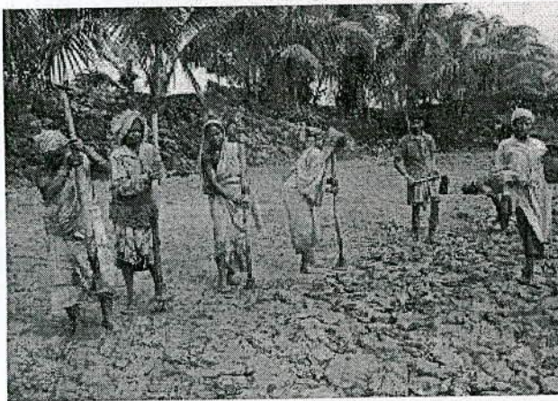
Figure 5.9 Compaction method of clay for CCL
