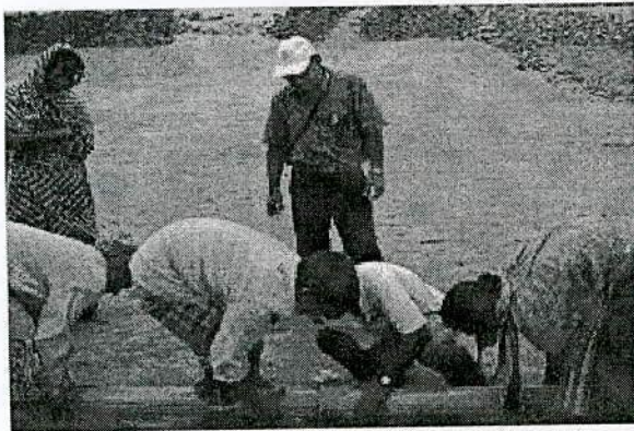
Figure 4.9 jointing of leachate collection pipe in the field
