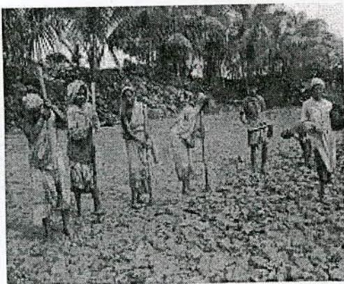
Figure 4.5 Manual compaction of clay to prepare CCL of the PSSL
