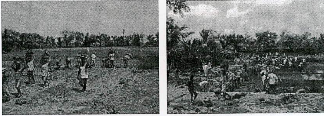
Figure 4.2 Manual excavation of earth using traditional digging tools
