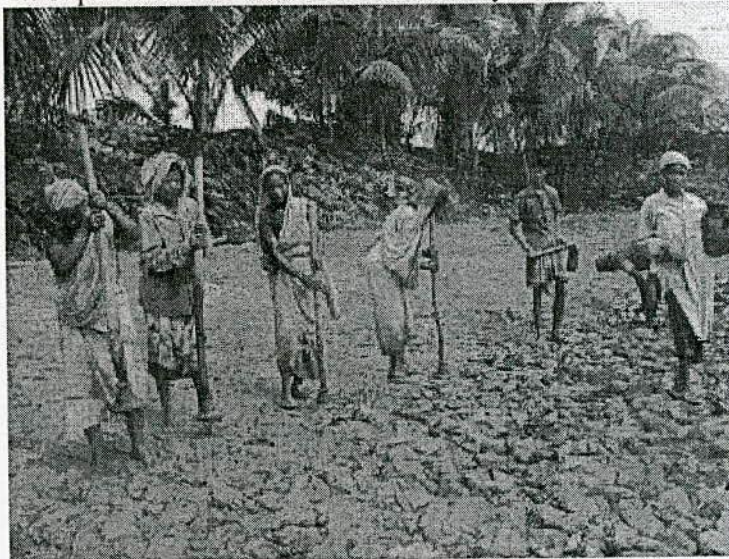
C- 5. Compaction of CCL at field, dated 12.05.08
