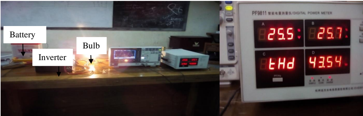
Figure 4.3: Total setup of harmonic analysis of a battery supplied inverter with load.
