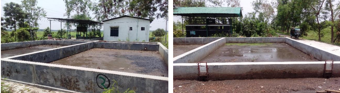
Figure 2.3: Sludge Drying Bed in Kushtia FSTP, Bangladesh (picture taken on May 16, 2017)
