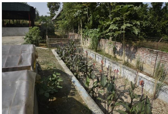
Figure 2.4: Typical Constructed Wetland in Shakipur FSTP, Tangail, Bangladesh. (Picture taken on 15 November, 2016)
