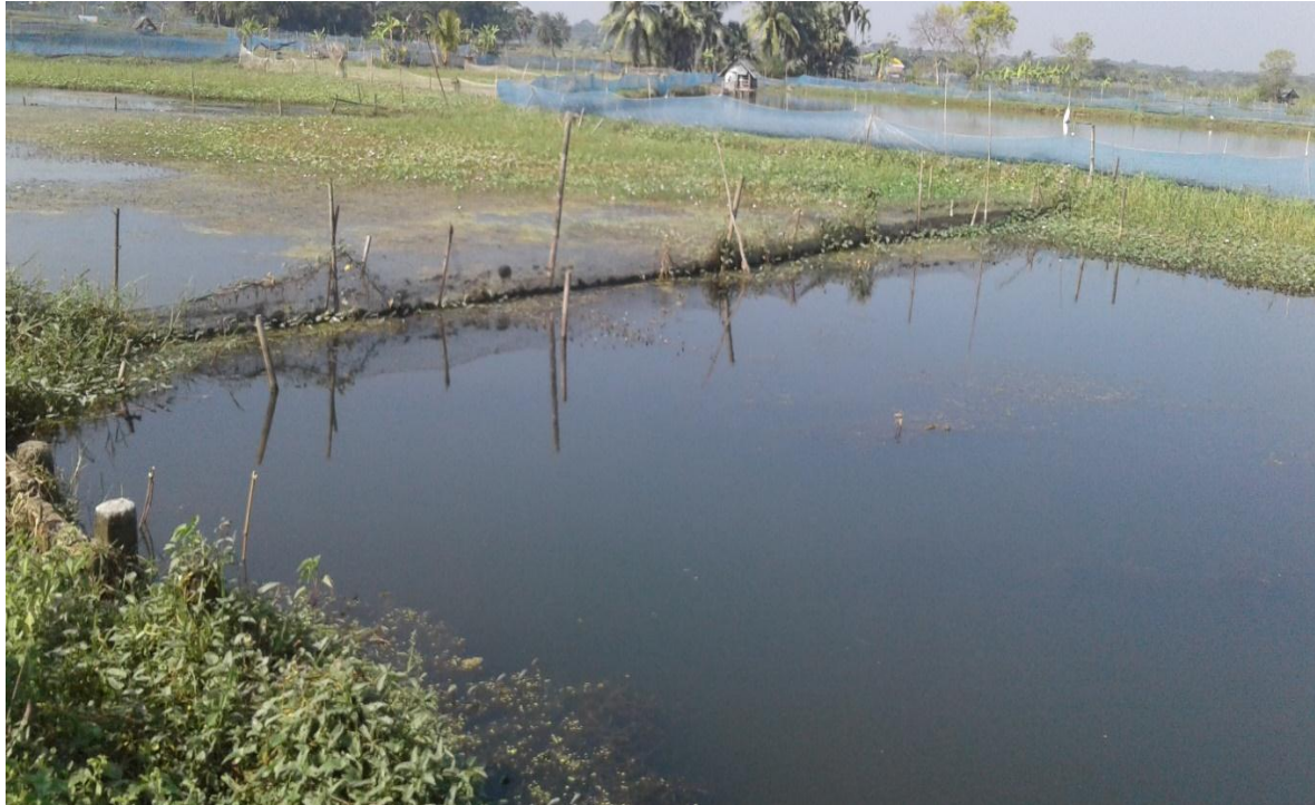
Figure 5.4: Blockage of drainage network due to fish culture.
