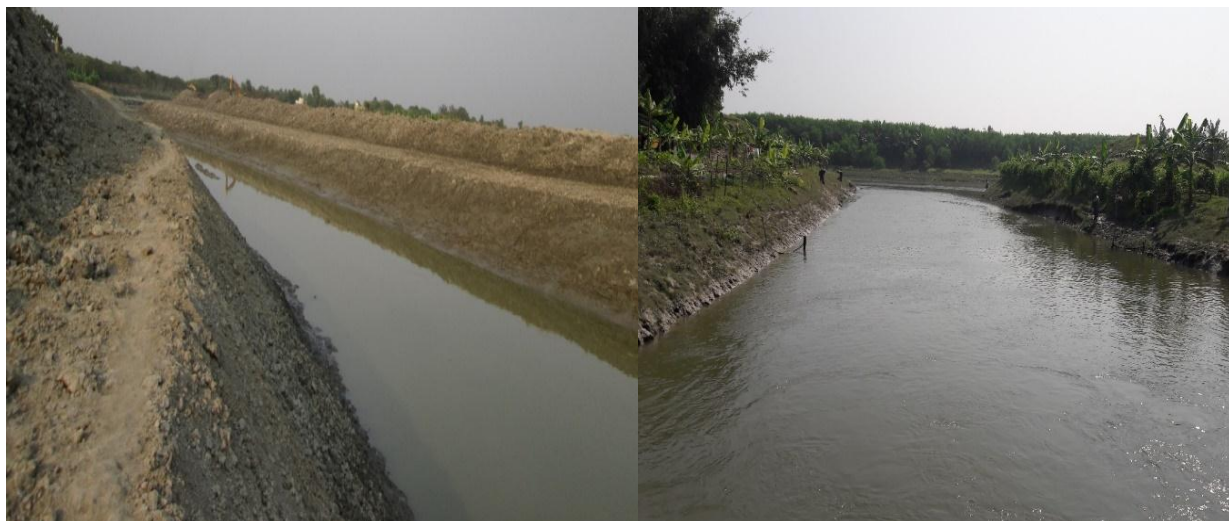
Figure 5.33: Improved situation of Kobadak river drainage system after completion of 2013-14 Financial year work (1st phase) dredging work of the river and canals.
