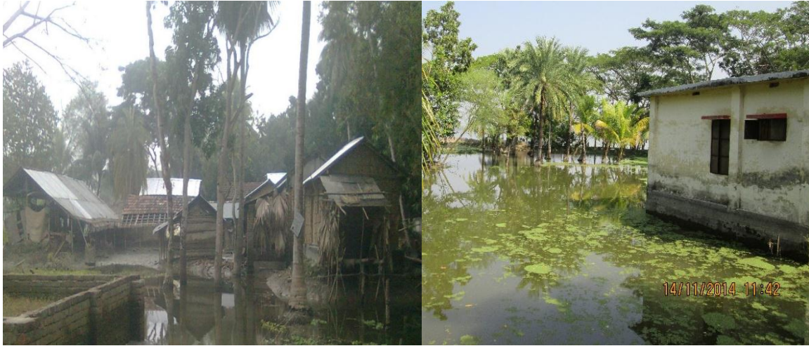
Figure 5.9: Damages of structure for water logging in the study area
