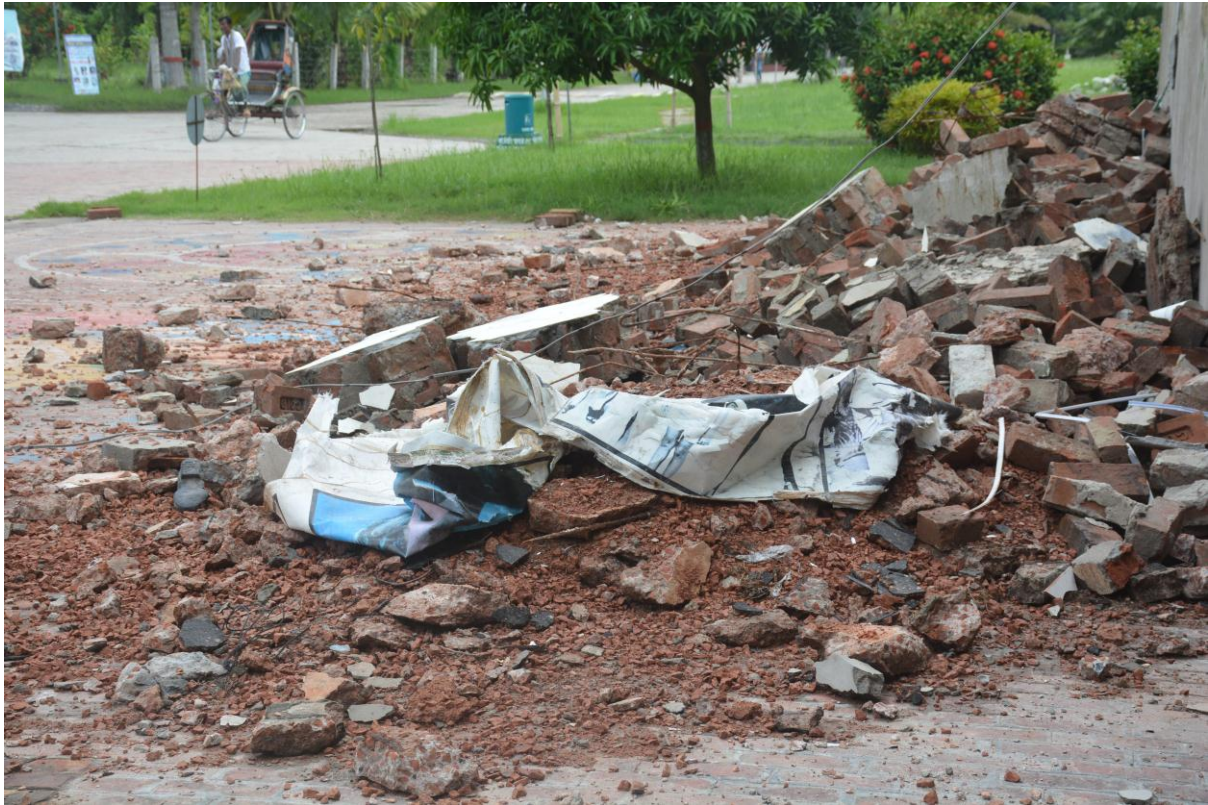
Figure 4.12: Destruction of Aesthetical View through construction Waste Deposition
