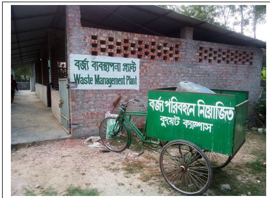
Figure 5.7: Solid Waste Management Plant in KUET
