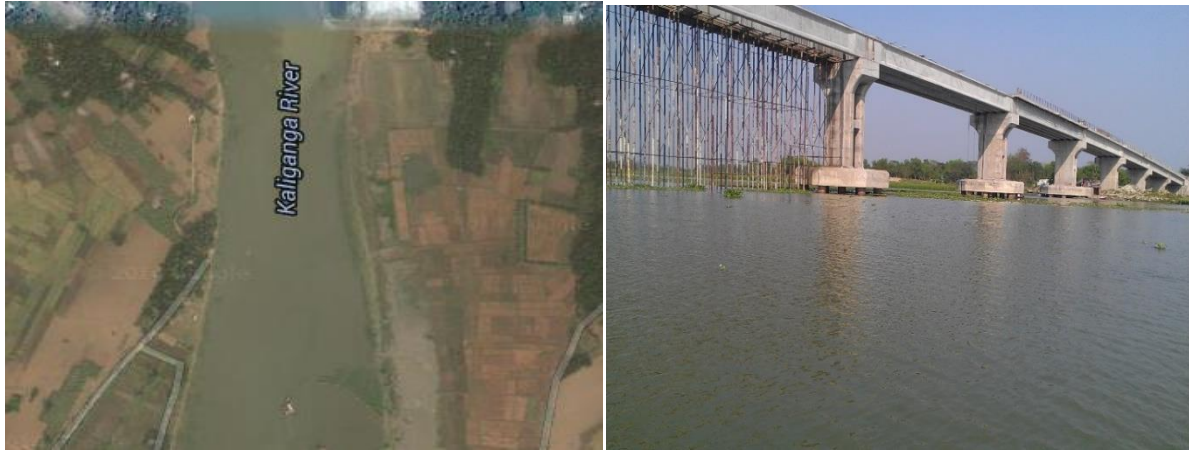
(c) Station 3: Chapailghat Bridge in Modhumoti River
